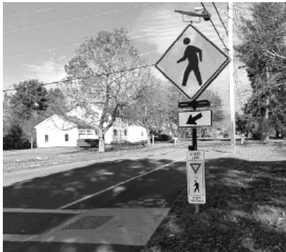
Typical Pedestrian Activated Crosswalk Warning Lights
