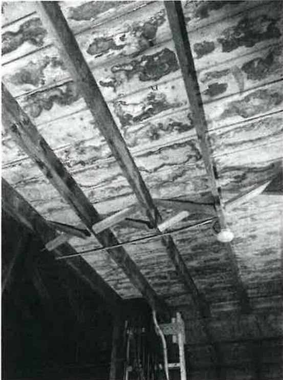
Photo 12: Detached diagonal blocking between joists
