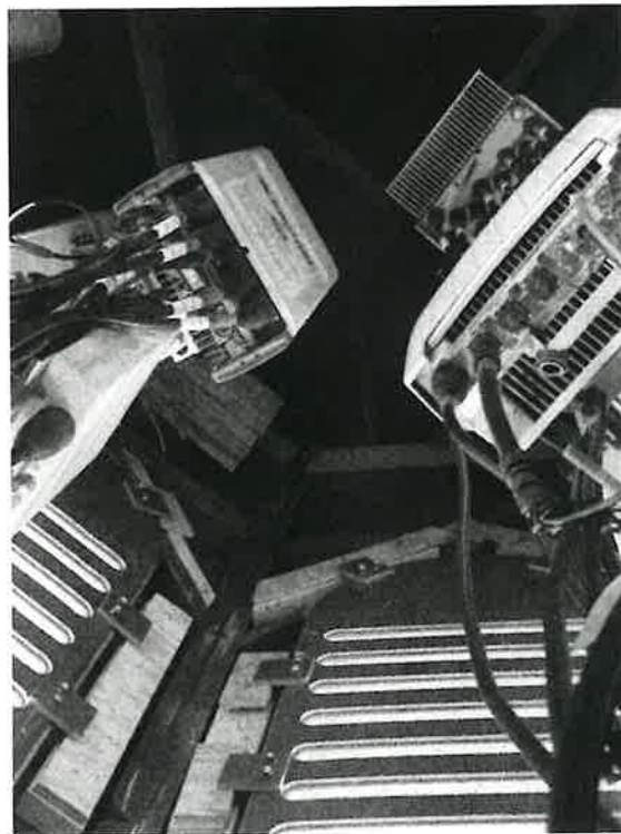
Photo 22: Cut original bracing and new wood "gusset plates"
