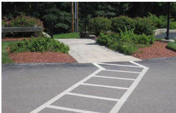
Clearly defined crosswalk
