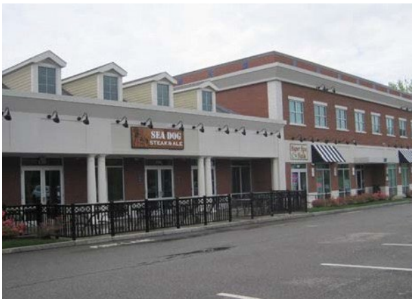
Mixing of building materials
