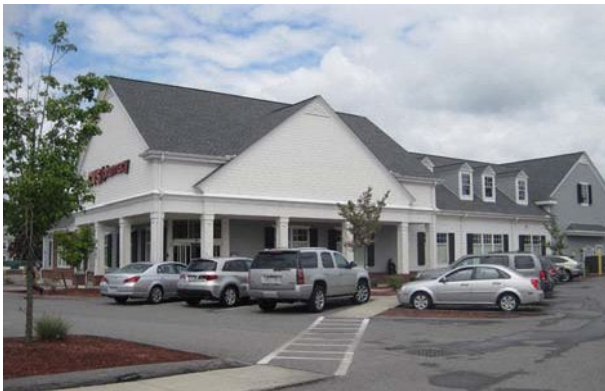
Detailed, articulated façade
