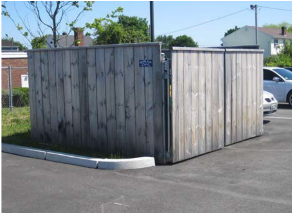
Example of appropriate utility screening
