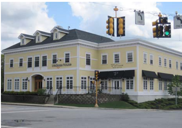
Large building visually reduced through design
