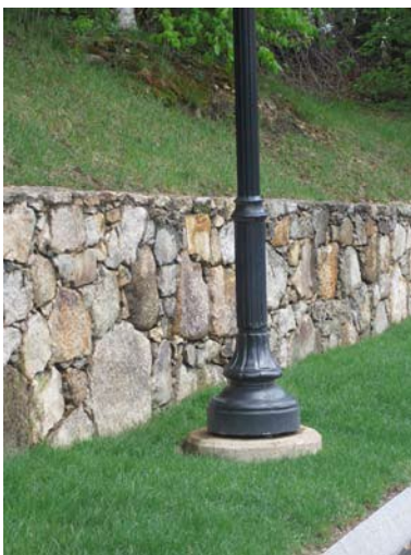
Correctly installed light post
