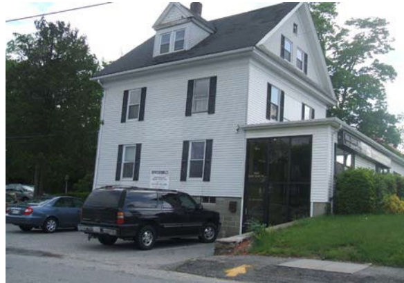
Building with undefined entrance oriented to parking lot
