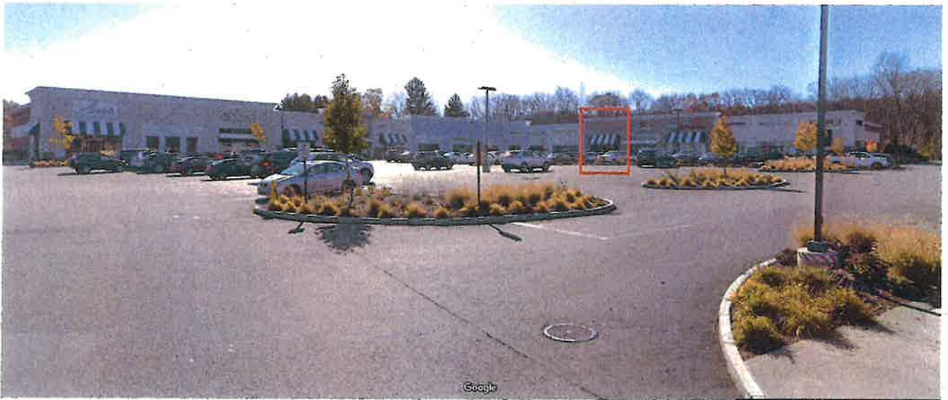
STREETVIEW - PARKING LOT ENTRANCE (TOP OF DRIVEWAY)
