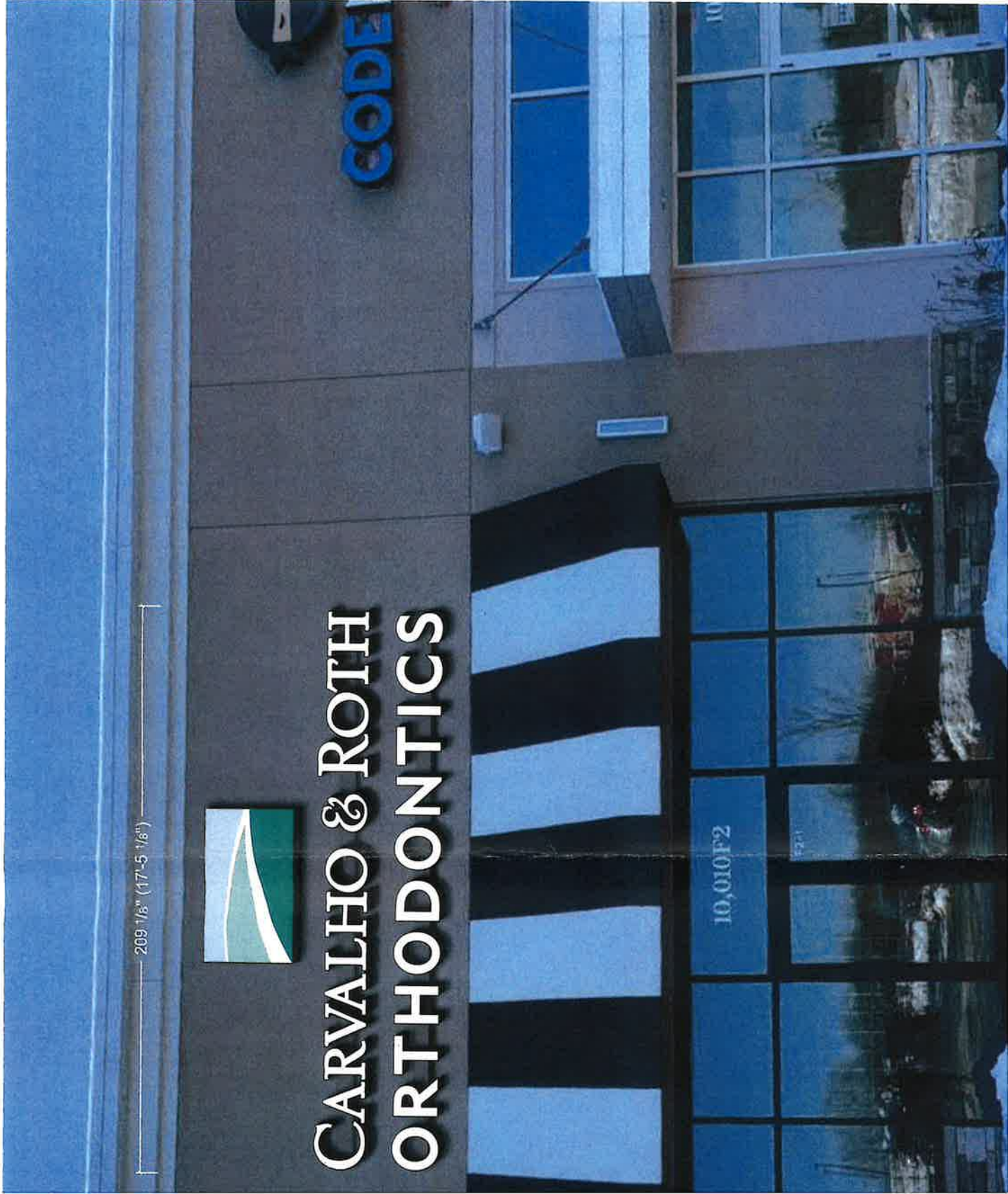
Ice-lit LED Channel Logo Icon & Letters Mounted to 5" Narrow Raceways
