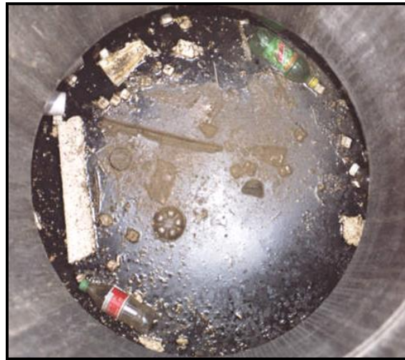
Floatable debris in the Aqua-Swirl ®
