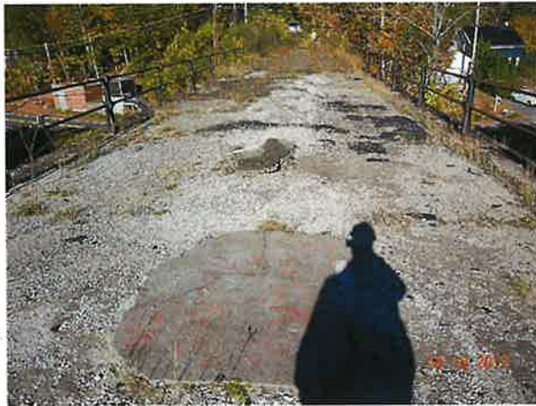
Photo 7: General Exterior View – Bridge Deck, Looking West
