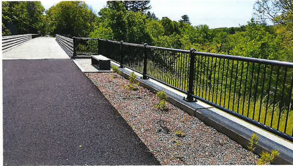
Figure G: Boston Pattern Railing (Foreground) on DCR Blackstone Greenway
