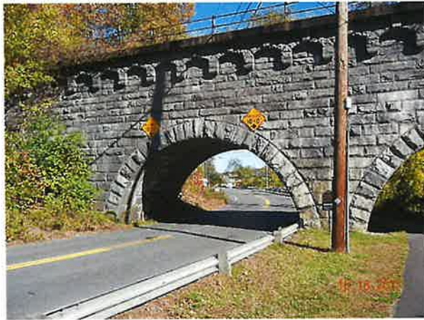
Photo 5: General Exterior View – South Elevation, Land Spans
