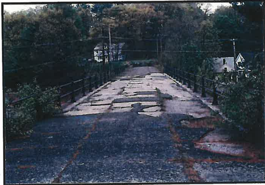
5. Deck Surface Looking West
