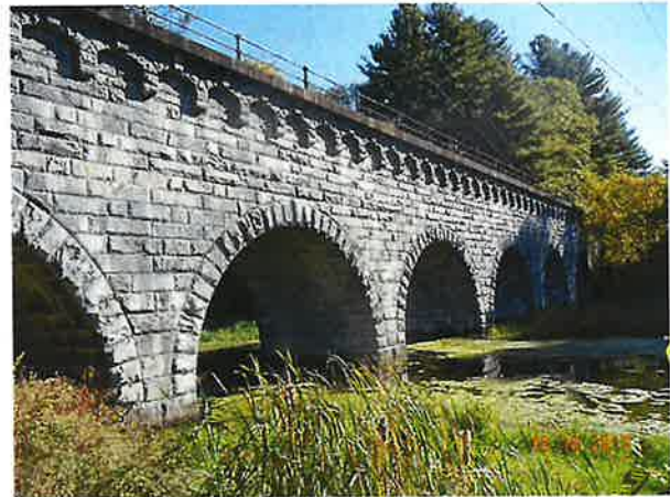
Photo 6: South Elevation, River Spans
