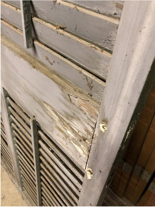
Close-ups of Damaged Shutters
