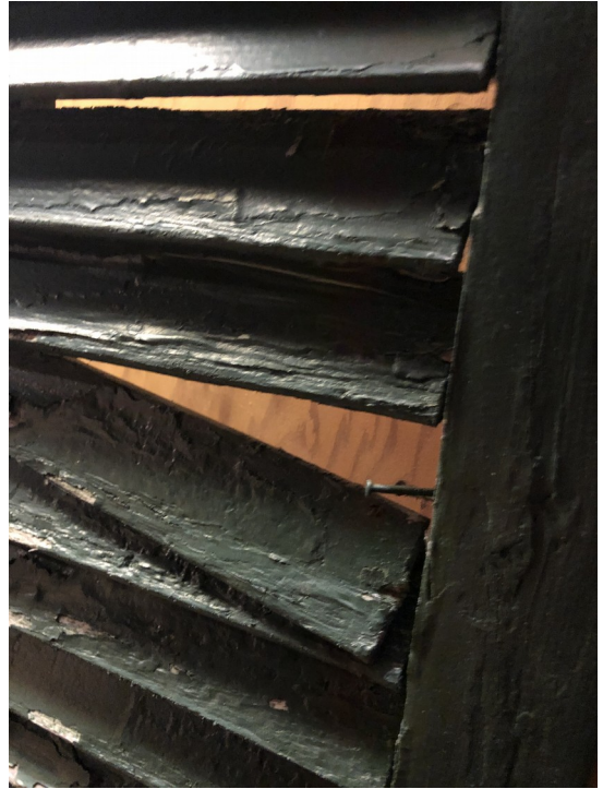
Close-ups of Damaged Shutters
