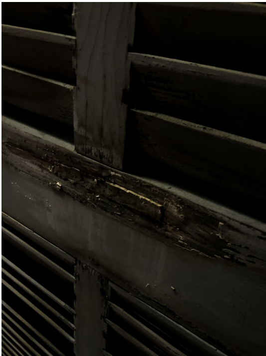
Close-ups of Damaged Shutters
