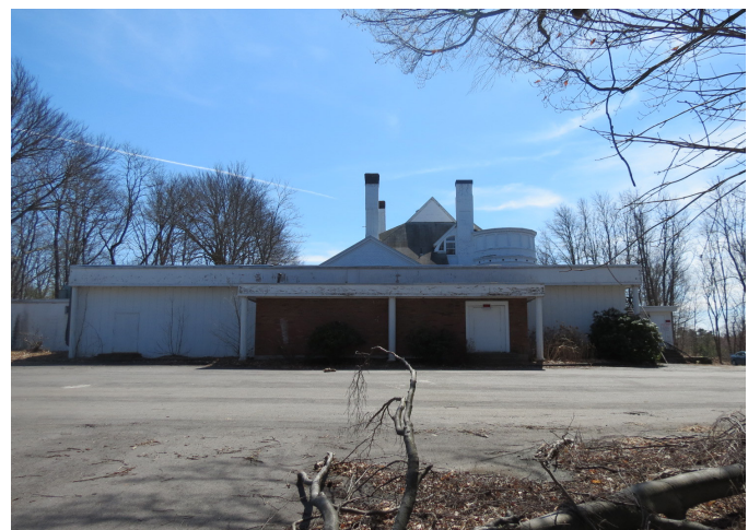
Figure 2.81: Exterior view of the ballroom addition.
