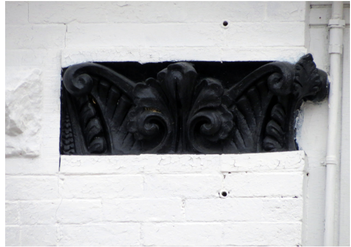
Figure 2.32: Terra cotta unit at the south facade
