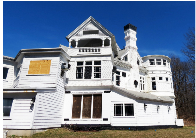
Figure 2.18: View from southwest depicting many window sizes and several removals.
