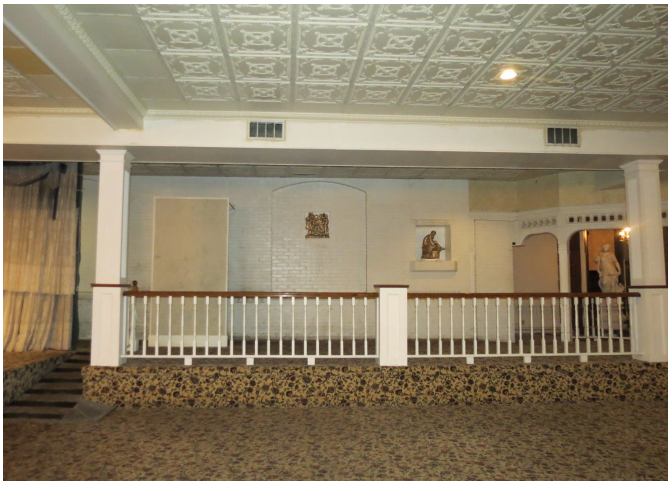
Figure 2.83: Original exterior masonry wall beyond.
