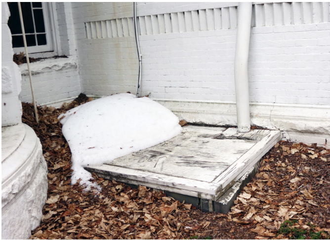
Figure 2.35: Exterior view of areaway adjacent to southeast turret.
