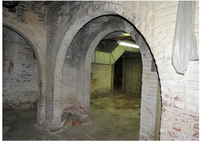
Figure 2.71: Typical brick masonry walls at basement.
