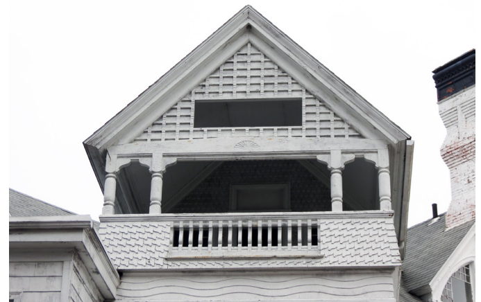
Figure 2.30: Third floor porch at west elevation.
