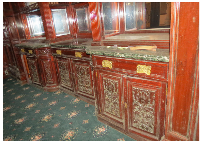
Figure 2.43: Surface build-up at hutch.
