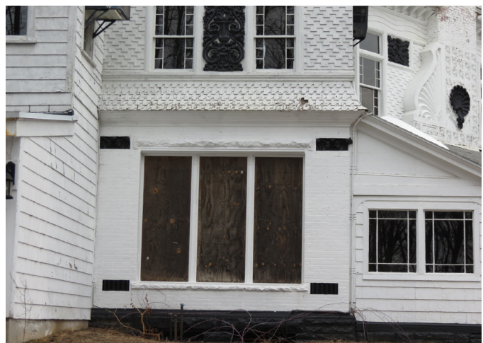
Figure 2.4: Brick masonry and brownstone foundation at southwest bay (painted).
