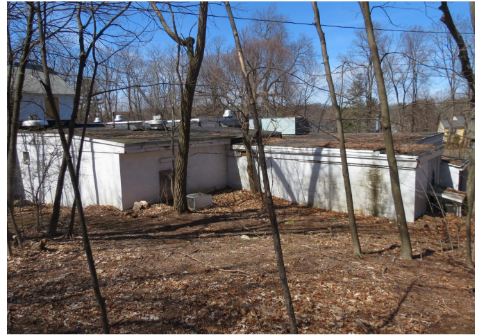
Figure 2.85: Exterior view of east addition.
