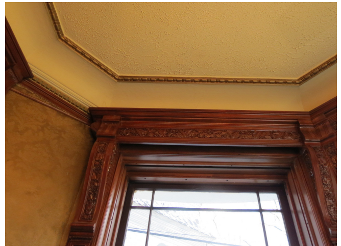
Figure 2.53: Simple plasterwork at southeast turret in Parlor.
