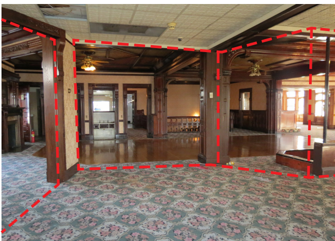
Figure 2.90: View from inside the second floor of the west addition toward the location of the removed exterior wall. Note the structural column in the right of the image.
