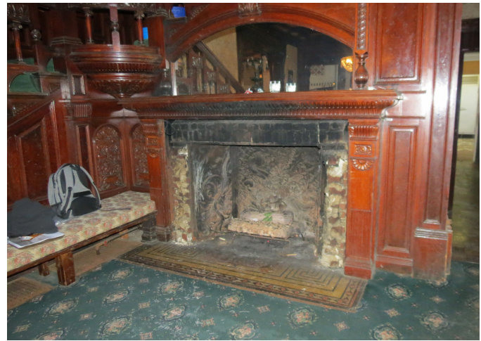
Figure 2.55: Fireplace at Entry Hall, note bronze surround has been salvaged.
