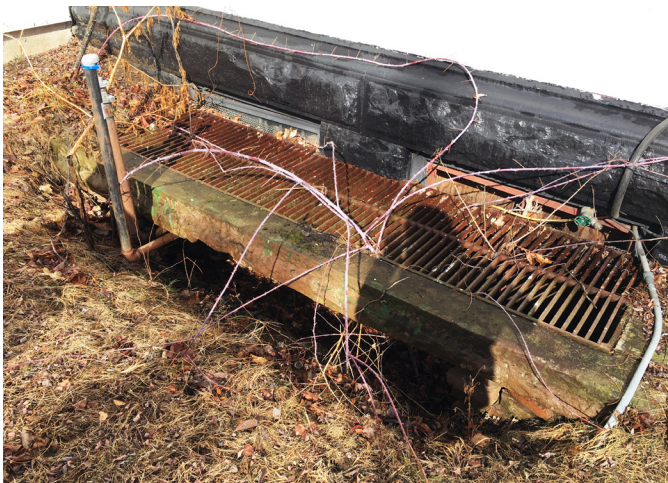
Figure 2.36: Exterior view of areaway at southwest bay.
