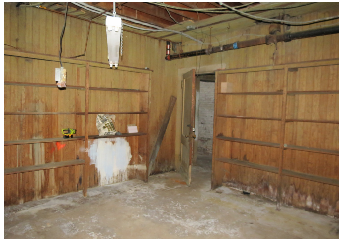
Figure 2.72: Wood paneled walls and ceiling at basement.
