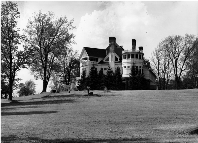
Figure 1.17: South elevation, 1946. Source: Northborough Historical Society.
