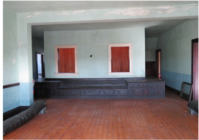
Figure 2.64: Light well at the third floor.
