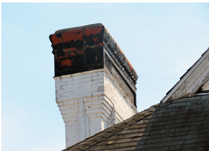
Figure 2.31: Terra cotta cap at the southeast chimney.
