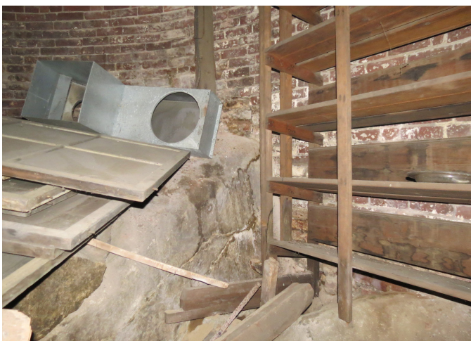
Figure 2.76: Wine cellar shelving built over ledge.
