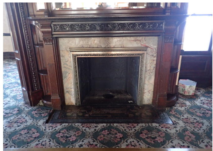
Figure 2.57: Fireplace at northwest corner of second floor.
