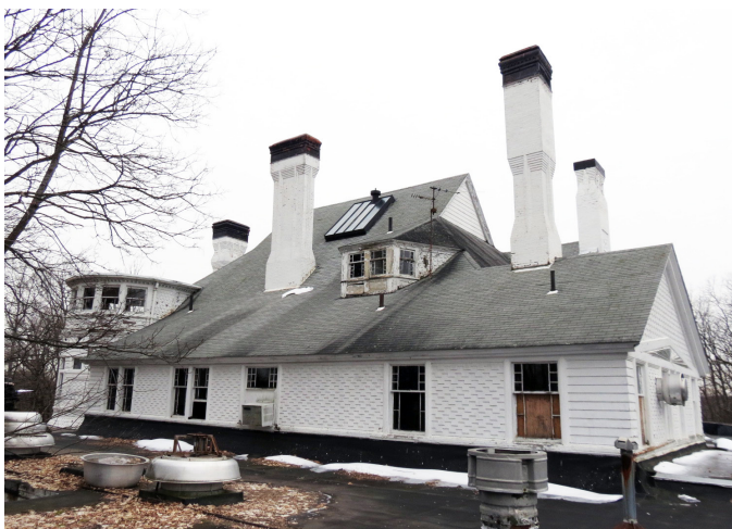
Figure 2.24: View from northeast partially depicting all chimneys.
