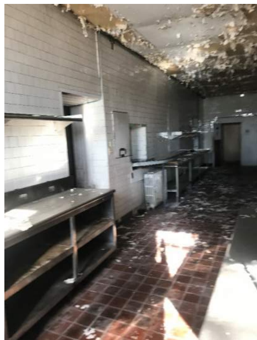
Electrical sub panel in the kitchen
