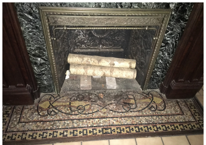
Figure 2.63: Detail view of fireplace in second floor multi-user restroom.
