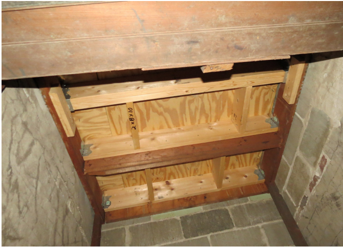
Figure 2.74: Enclosure at original exterior basement stair.
